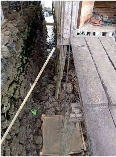
Base of a cement stilt.
